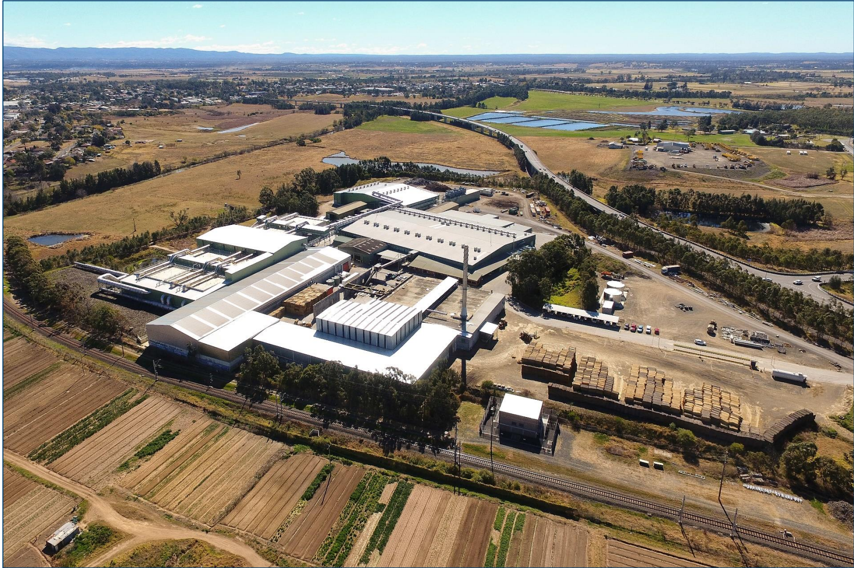
Figure 2-1: Completed MOD1 Project
