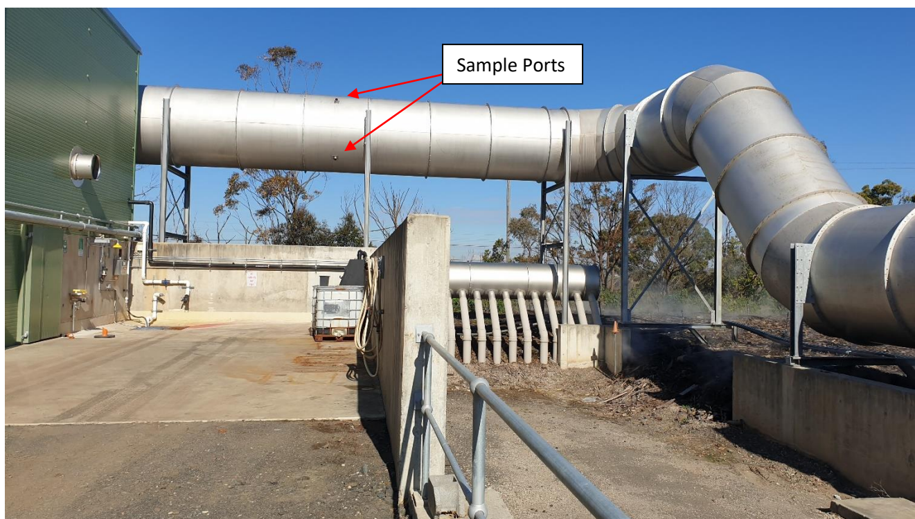
Figure 4 Illustration of Western Biofilter Inlet Sample Ports
