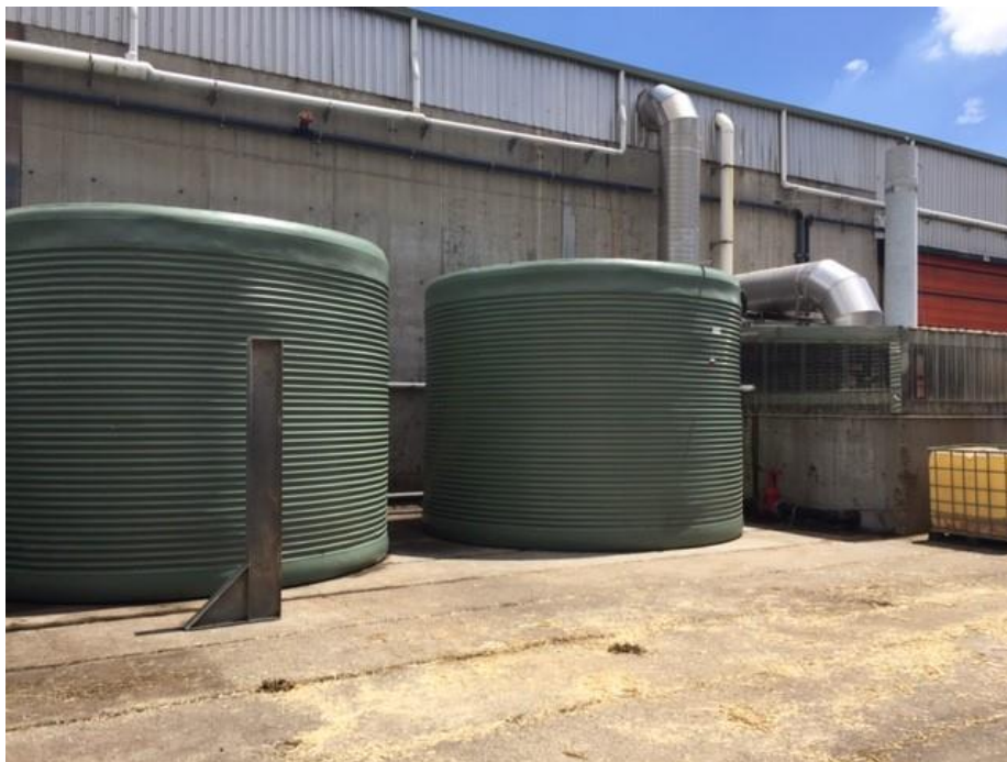
Photo 8 Two Additional Balance Tanks when La Nino Event Predicted
