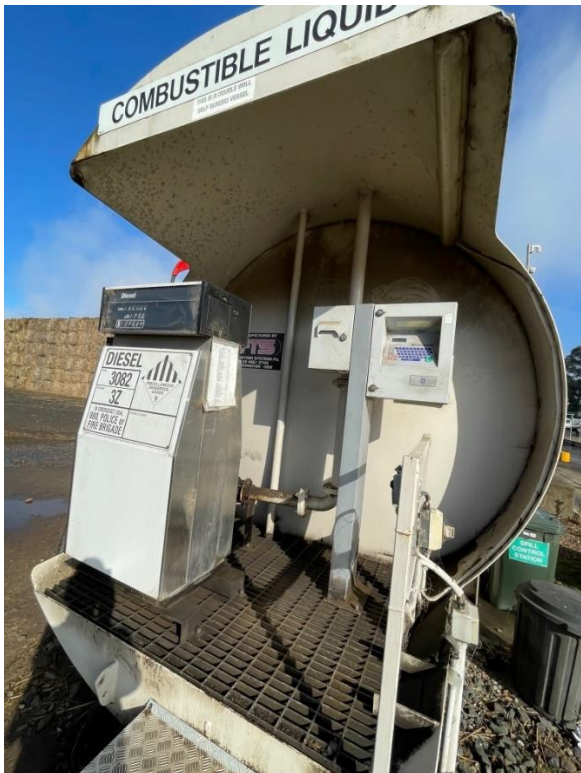
Photo 12 Double Skin Storage and Spill Kit
