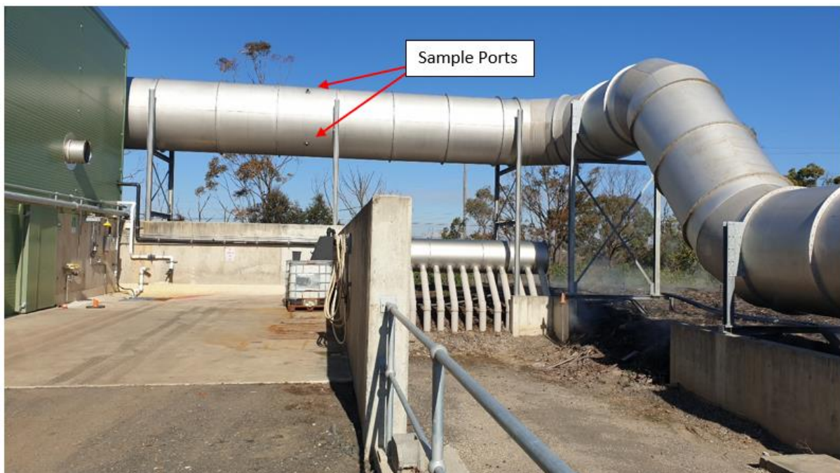
Figure 4 Illustration of Western Biofilter Inlet Sample Ports
