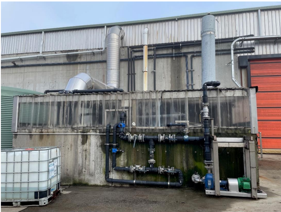
Photo 6 Enclosed Wastewater Pit
