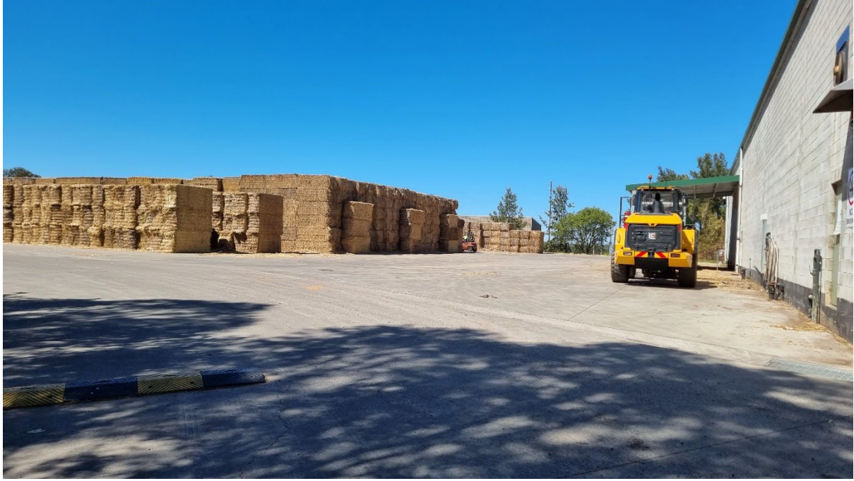
Figure 1 Bale noise wall and fire separation from building - October 2023
