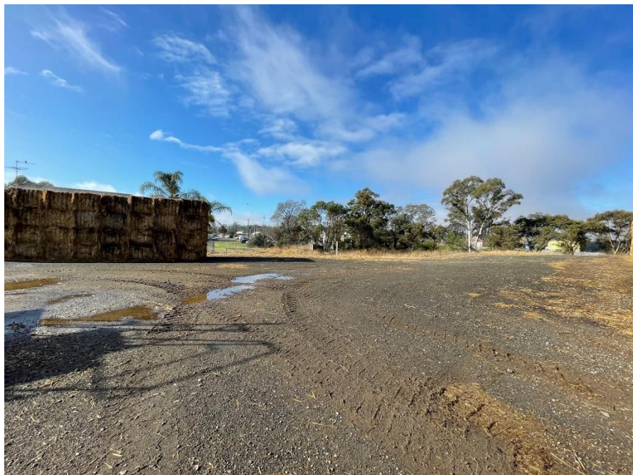
Photo 14 Temporary Noise Barrier
