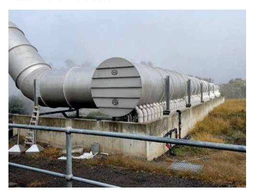
Photo 4 Biofilter – Upper Section
