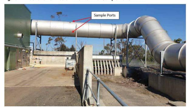
Figure 5 Illustration of Eastern Biofilter Inlet Sample Port
