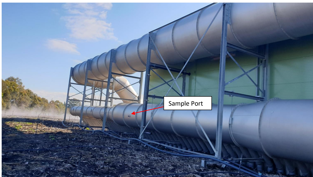
Figure 5 Illustration of Eastern Biofilter Inlet Sample Port
