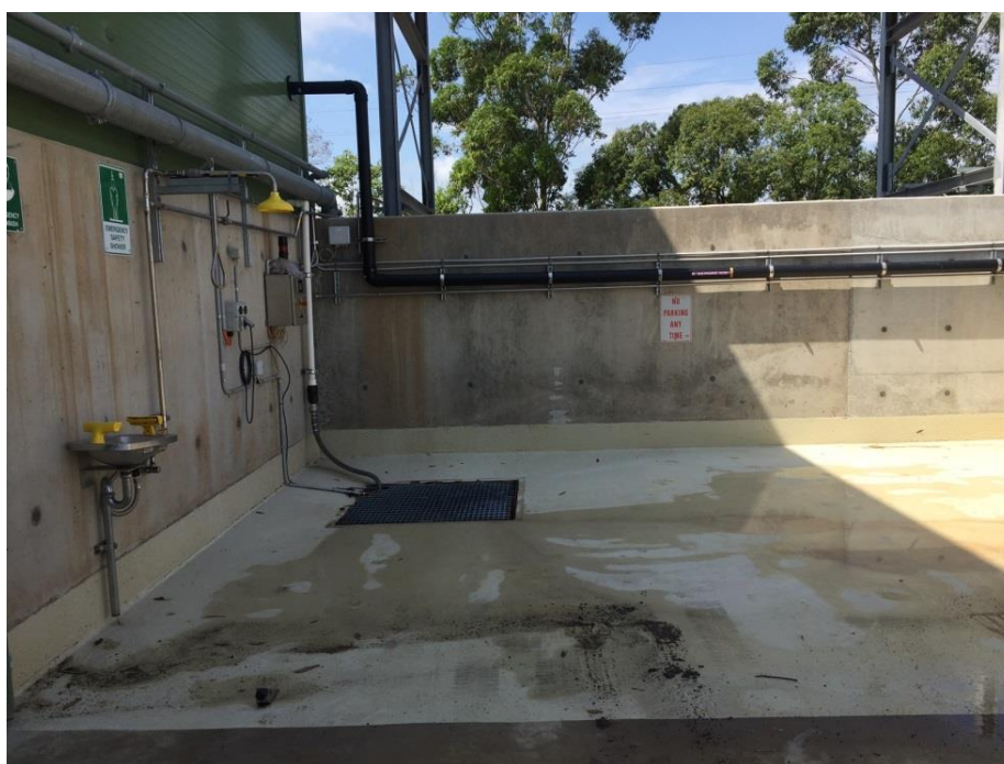
Photo 6 Emergency Shower and Drainage to Capture Spills from Unloading
