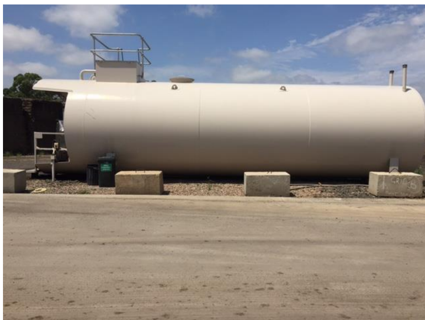
Photo 14 Diesel Fuel Storage – Double Skin
