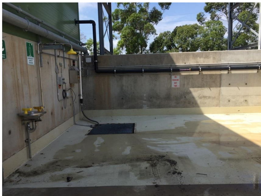
Photo 6 Emergency Shower and Drainage to Capture Spills from Unloading
