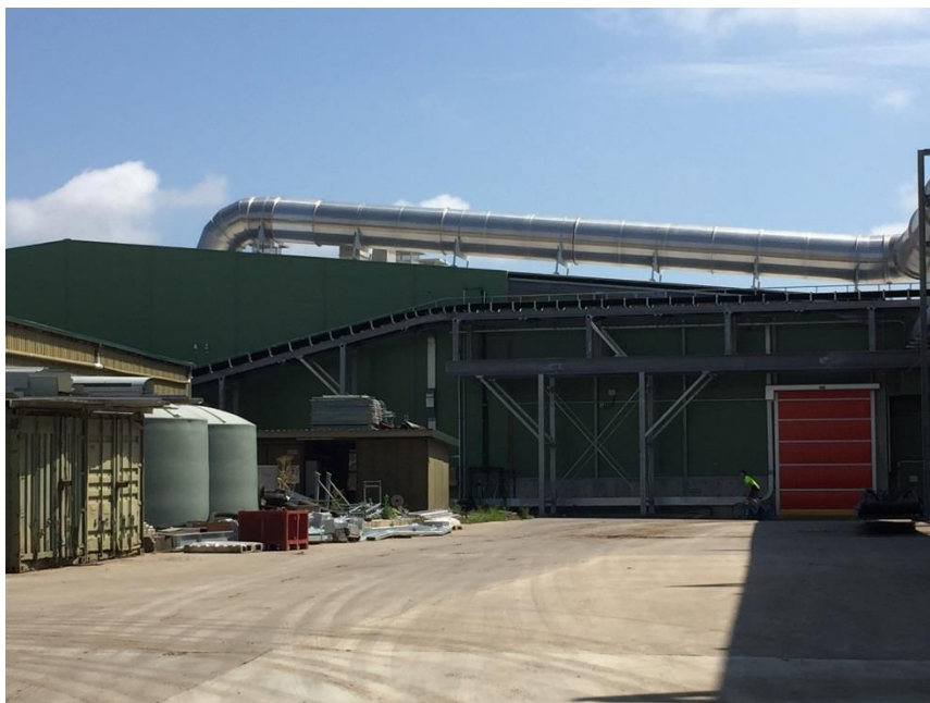
Photo 1 New Plant – Construction Completed – Shows Ductwork for Transferring Process Air to the Odour Control System
