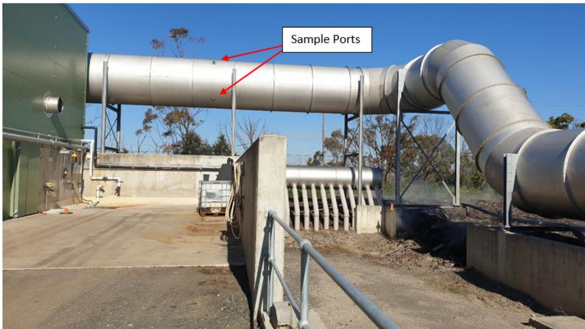
Figure 4 Illustration of Western Biofilter Inlet Sample Ports
