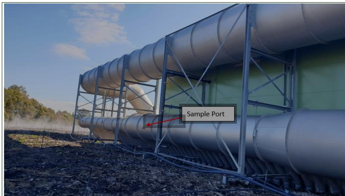
Figure 5 Illustration of Eastern Biofilter Inlet Sample Port
