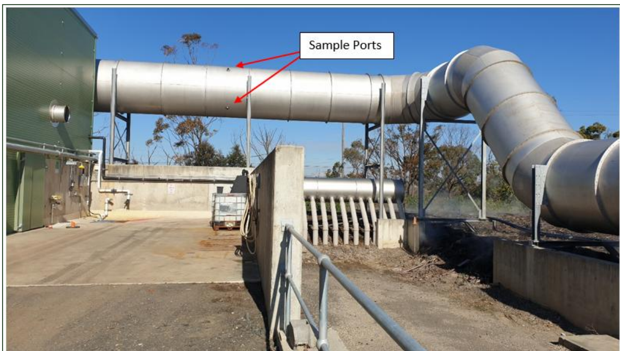
Figure 4 Illustration of Western Biofilter Inlet Sample Ports
