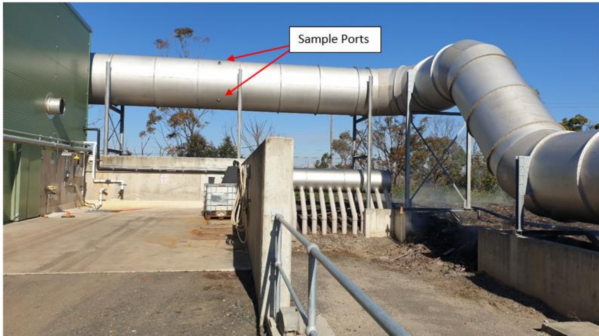
Figure 5 Illustration of Eastern Biofilter Inlet Sample Port
