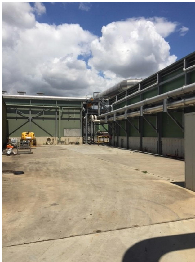
Photo 1 General plant area including Ductwork for Transferring Process Air to the Odour Control System
