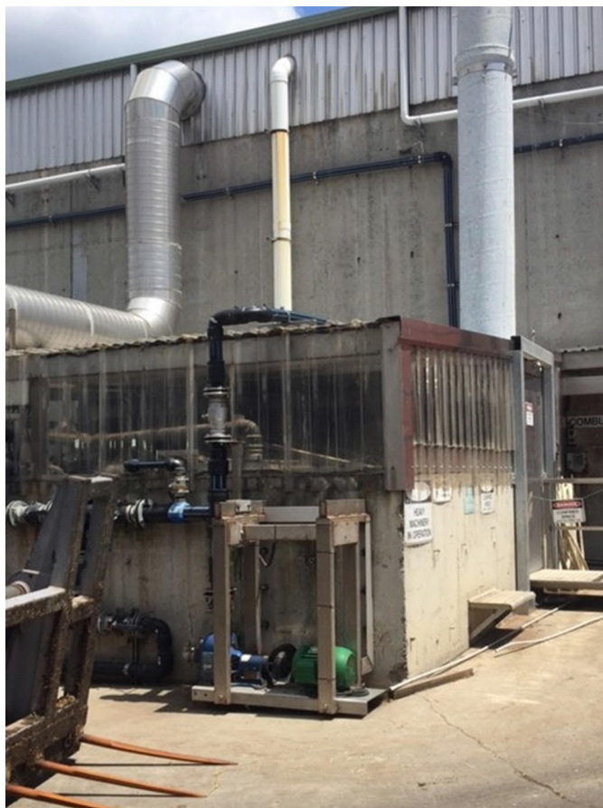
Photo 6 Emergency Shower and Drainage to Capture Spills from Unloading
