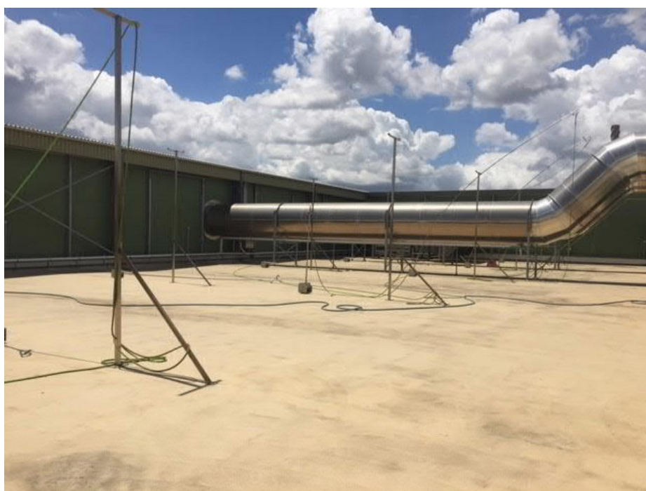
Photo 2 Ducting to Biofilter from Process Area
